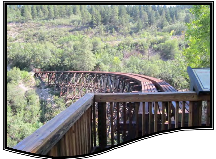
View from the southern viewing area of the Mexican Canyon Trestle
